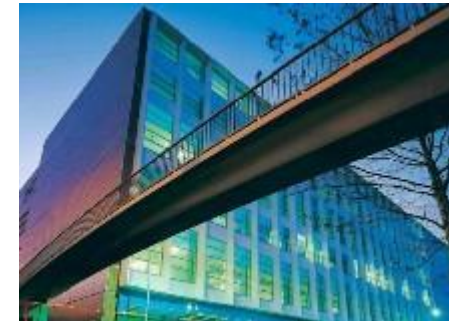
Data centre at Global Switch housing our servers and 2 100mb internet links
